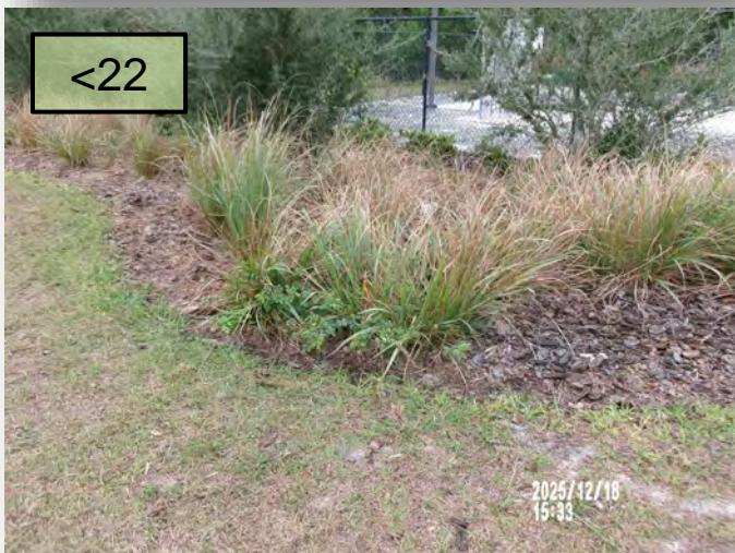
24. Along Pond D, one of the drip lines from a removed tree is still running. Please have the irrigation team cap off this line until further notice, the line is causing an erosion spot. (Pic 24>)
